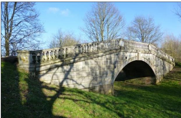
L. Portland stone bridge by Sir William Chambers
