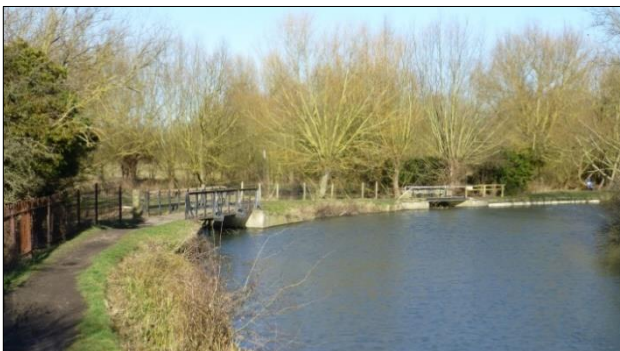
J. Sluice gates and weir on the River Stort
