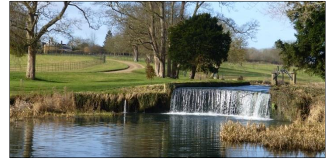
C. The sluice gate, cascade and tumbling bay
