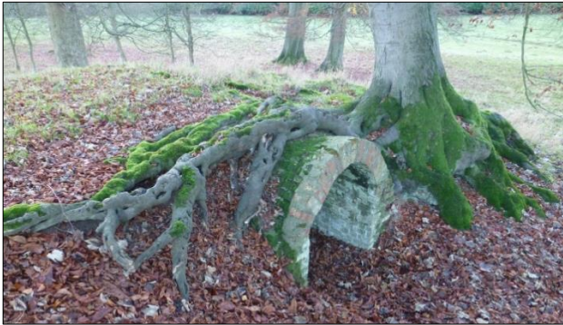
B. Ice house earthen mound and vaulted tunnel
